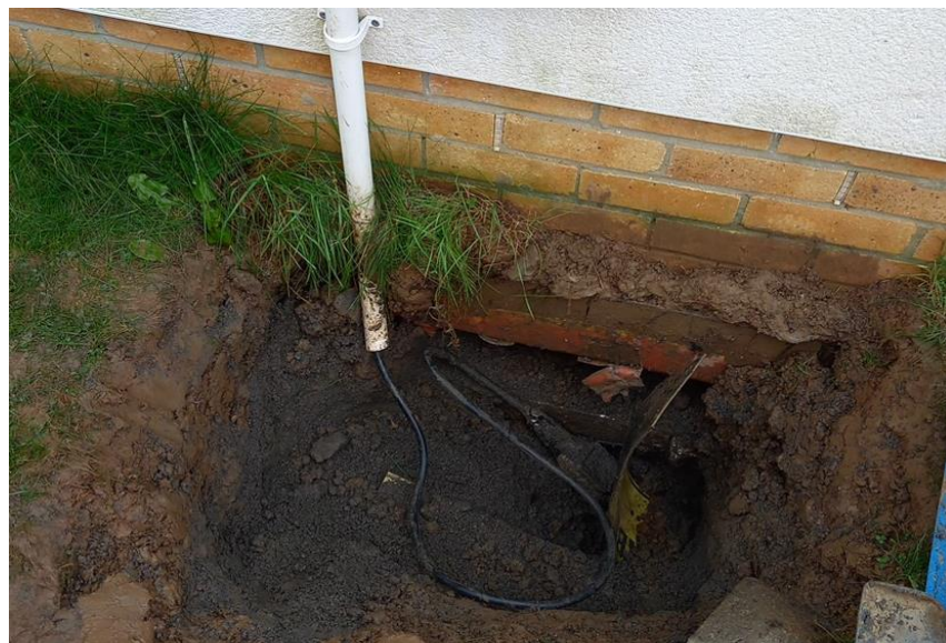
Figure 2: Service joint and coil of 35mm 2 service cable.
